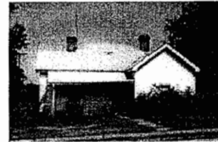
New South Cottage
