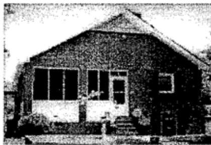
Brick veneer has been inappropriately added to this originally wood-sided house.
