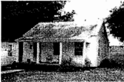
Several variations of porches are found on the side-gabled houses of Beaumont, including this shed porch.
