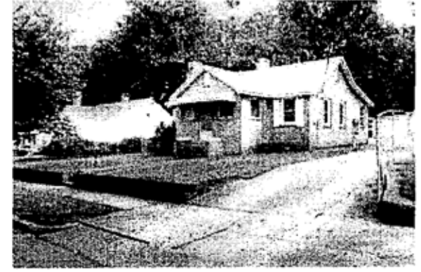
Retaining Wall example within the district.
