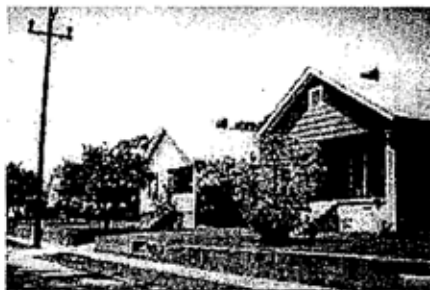
These front-gabled roof forms help define these house types.
