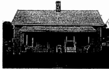
This house originally had two front doors, but one has been completely removed, changing an important character-defining feature of the house.
