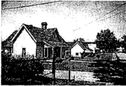
The one-story height of these saddlebag houses is a characteristic element of the type.
