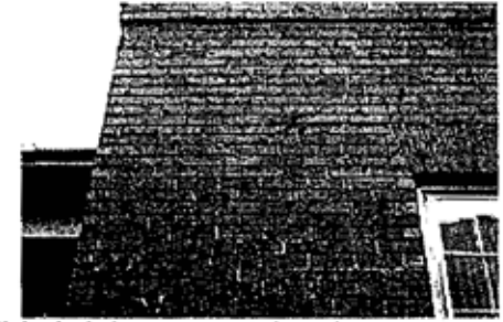
This brick masonry has been properly maintained.
