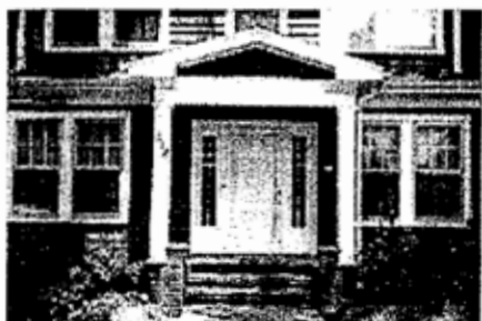
The square posts, low-pitched pediment, and multi-paned sidelights of this entrance are distinctive features of the Craftsman style that should remain intact.
