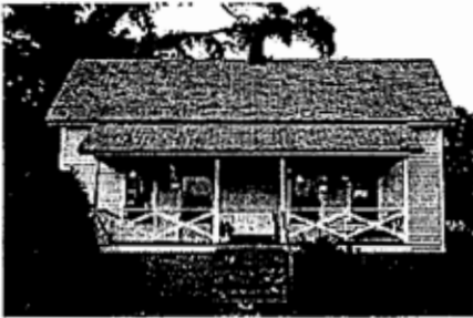
This saddlebag retains its original two front doors.
