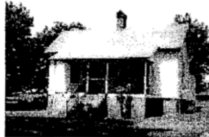
The central chimney is the most significant feature in the definition of the saddlebag house type.
