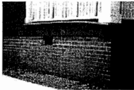
This solid brick foundation is in good condition.
