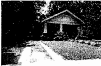
Photograph illustrates an example of "driveway tracks" or driving lanes, a historic treatment that should be retained.
