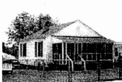
This front porch has been enclosed with screen, maintaining its original open character.
