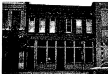
Reconstructed but compatible wood storefront.
