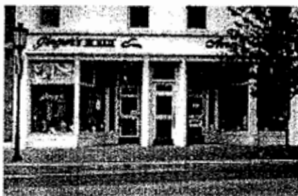
Intact storefront with cast-iron columns, recessed entry, large display windows, and transom windows.
