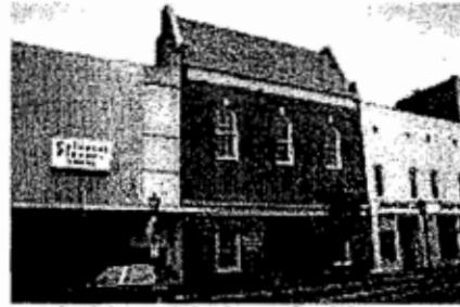
Unusual side-gabled roof with parapets.
