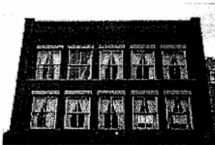
Open and well-maintained upper-floor windows and details.
