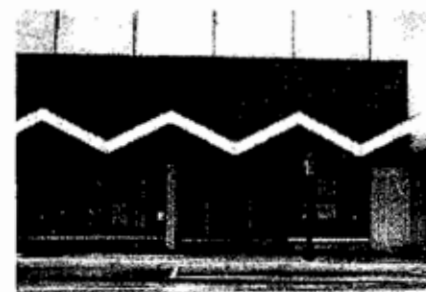
Example of incompatible awning design and material.
