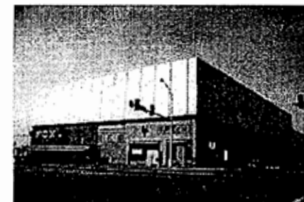
Original storefront elements may exist under nonhistoric material and should be uncovered.
