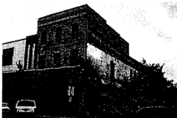
Vacant commercial building that has been neglected.
