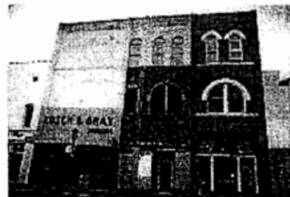
Infilled window openings that are now being reopened.
