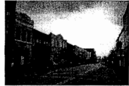
Typical flat roofs with parapets.
